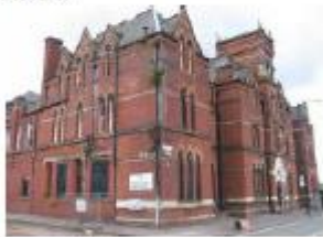
North East corner 2004
